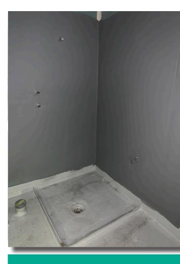
Low Odour, Low VOC, Modified Acrylic Waterproofing Membrane with Micro Fibres
