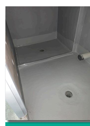
One Part, Single Coat Application, Polyurethane Waterproofing Membrane
